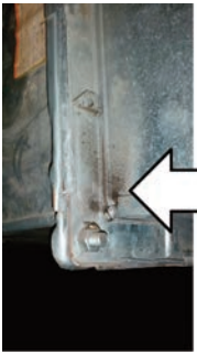
Tracing at corners of flanges
